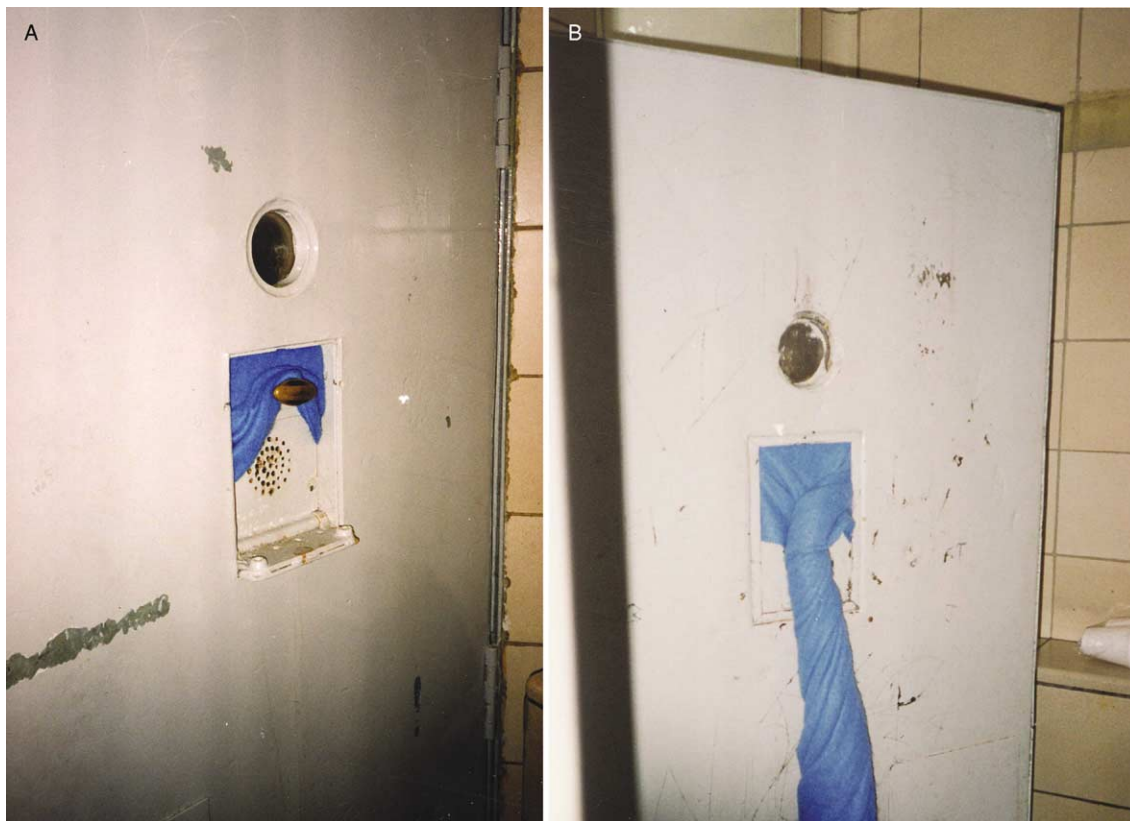
Figure 1 (A) The view of the “wicket,” which had previously been left open for a prisoner. The blue is a blanket that has been wrapped around the wicket, which was then pulled shut from within the cell. (B) The view from within the cell, demonstrating how the prisoner had used the cell blanket in an attempt to self-harm, by twisting it around his neck, and allowing suspension from the wicket.
