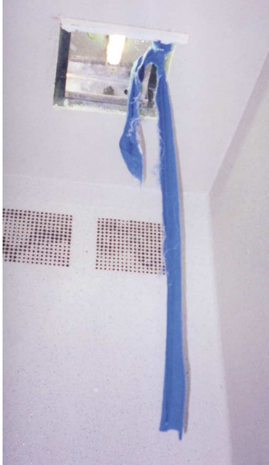
Figure 2 Broken recessed lighting panel; the sharp edges were used to cut the cell blanket into strips, and the light surround was used as a suspension point.
